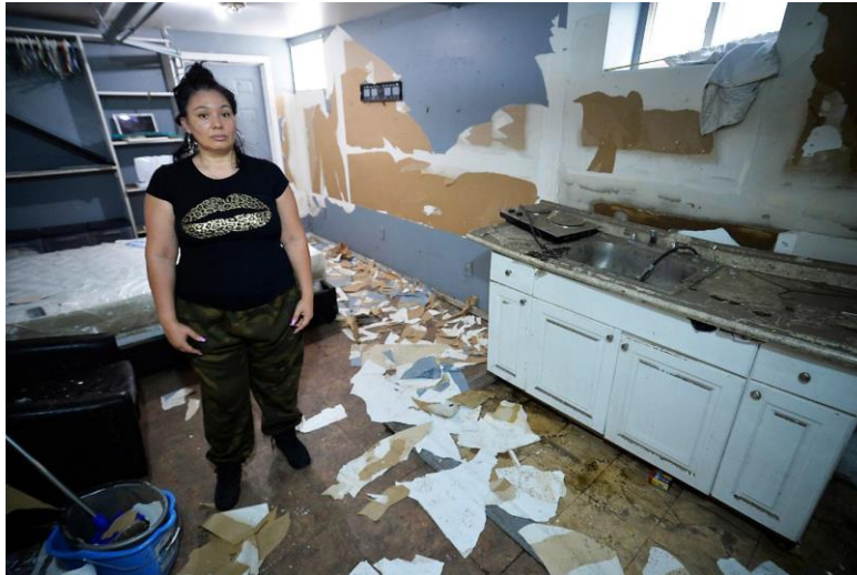
Hurricane Ida basement flooding
